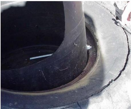
Photo 3. Start the nut on the rod outside of the tire and then slip it inside to thread the rod into the tire
